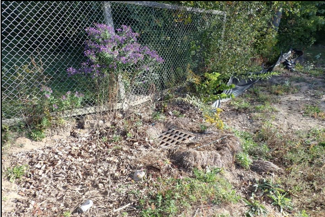
Photograph 10. Pond Spring Outflow to a Stormwater Catch Basin (September 2025)
