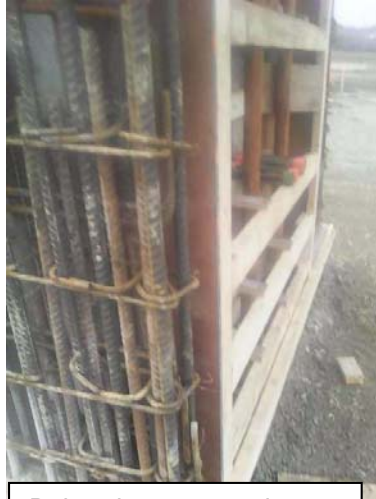
Rebar that structural guy wanted added
