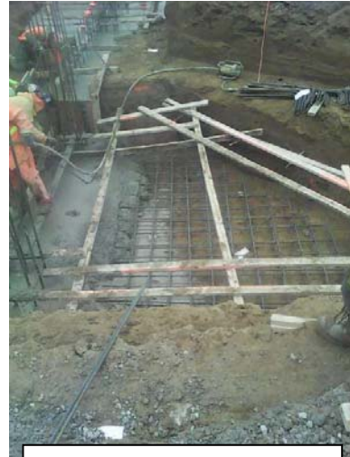
Rebar Ice Melting Pit Slab A-line
