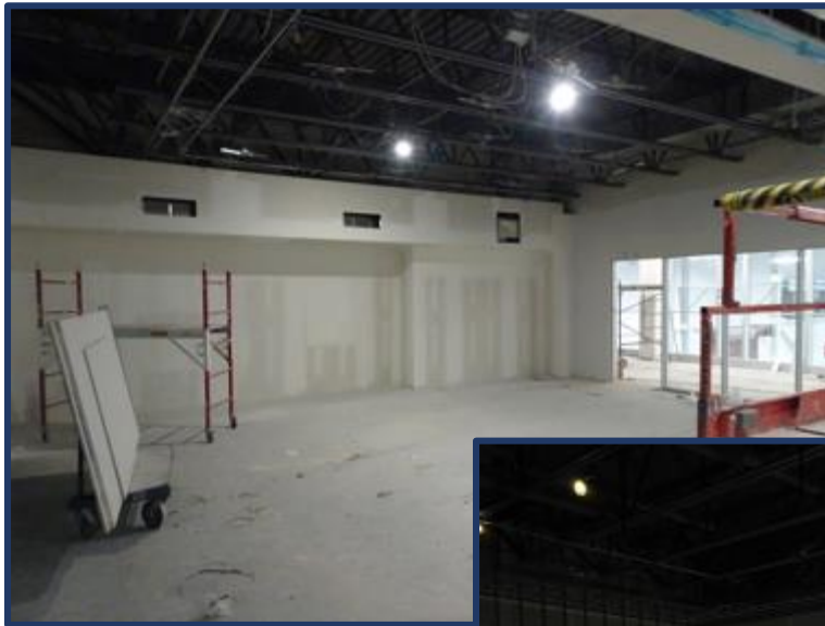
↑ 2 nd Floor Public Meeting Room
