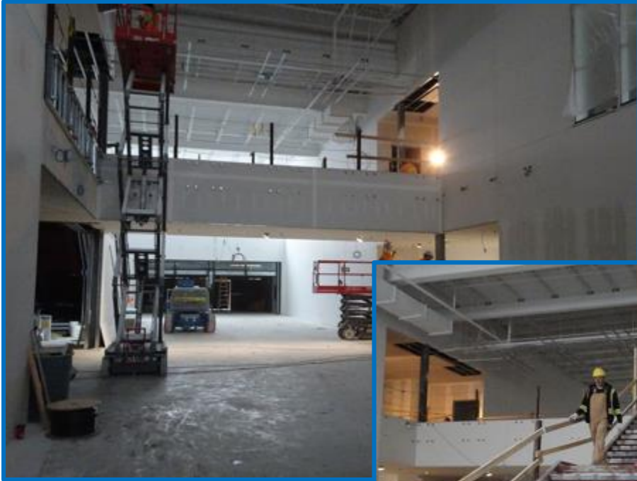
↑ Main Foyer Looking South
