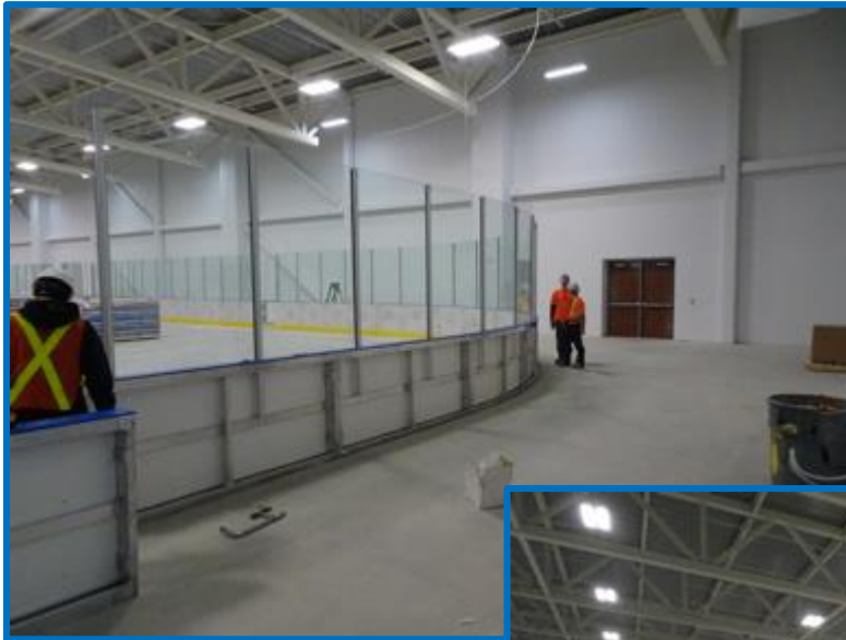
Rink B Boards Being Installed
